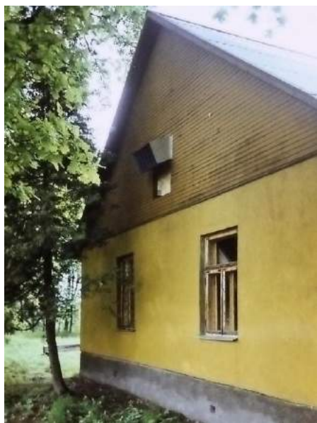
Air intake in the Sepa farmhouse
